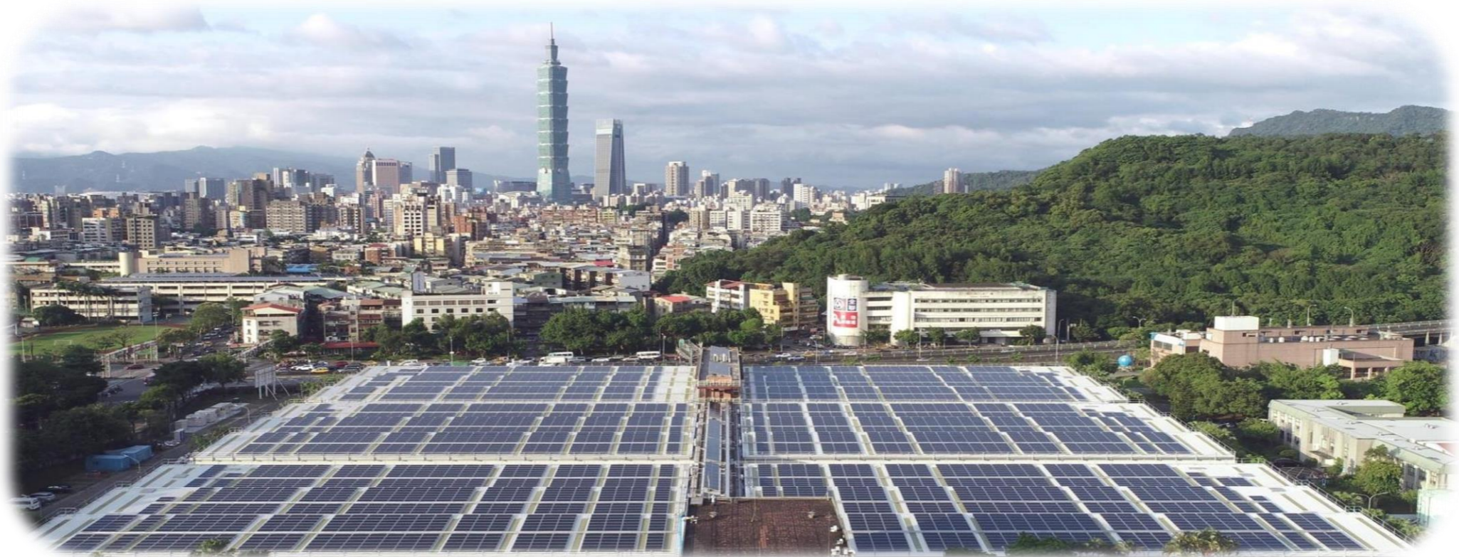
Taipei Water Department Chanxing Water Purification Plant
